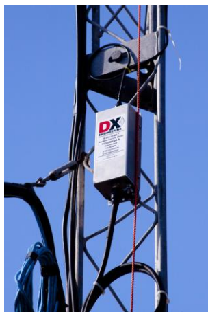
Feed Line Current Choke
